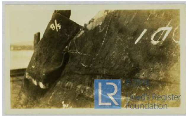
31- Close up photo of Fullagar's metal plate damage after the 1930 crash
